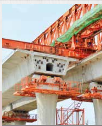
Precast Segmentation Box
