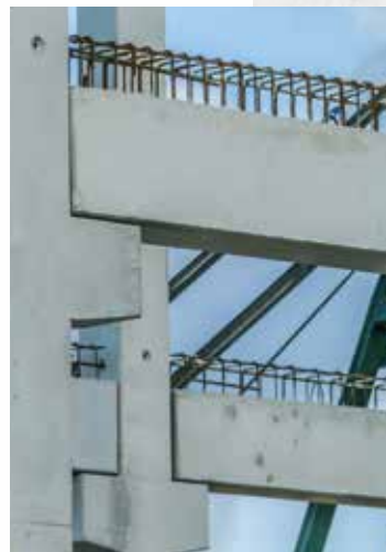
Beam & Column (Precast Building)
