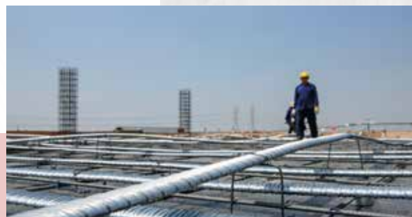
Bonded Post Tension (Flooring)
